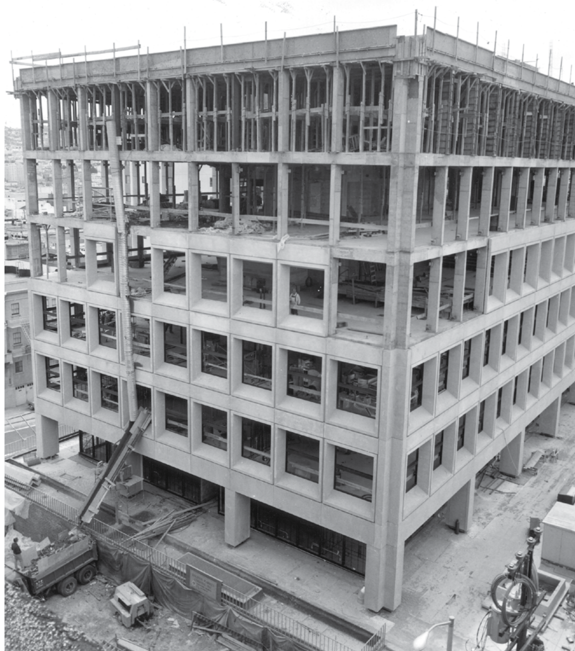
The facade is almost in place on the "new" dental school in this 1966 photo.
